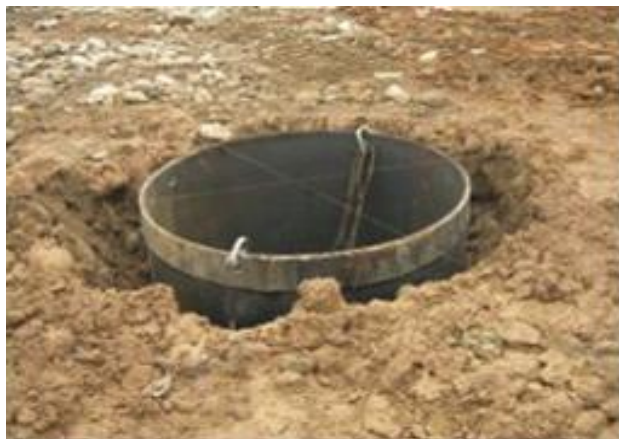
钻孔钢护筒埋设
